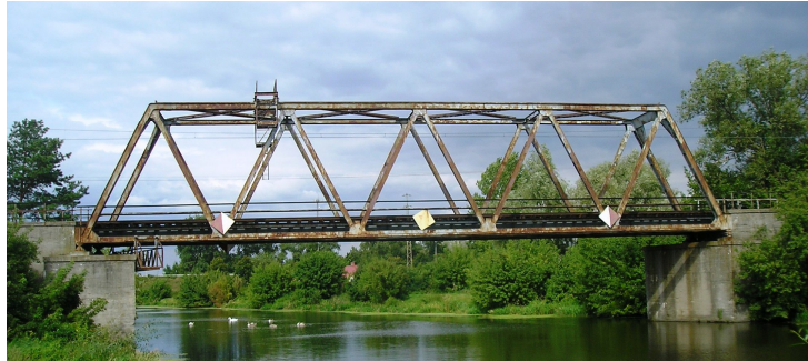
Fig. 1 Investigated railway truss bridge in Nieporet
